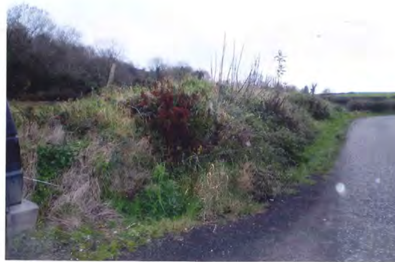
PHOTO SHOWING EXISTING VERGE / DITCH - N°1
