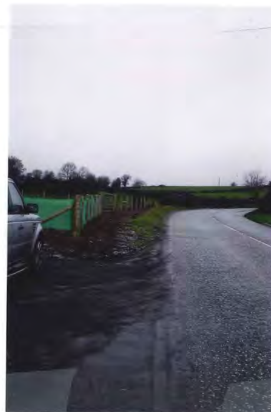
PHOTO SHOWING VISIBILITY SPLAY IN PLACE.
