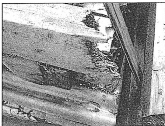
Damaged and decayed end of vertical timber member.
