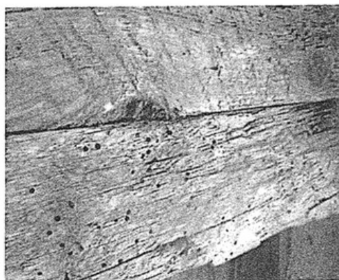
Woodworm/beetle infestation to timber.
