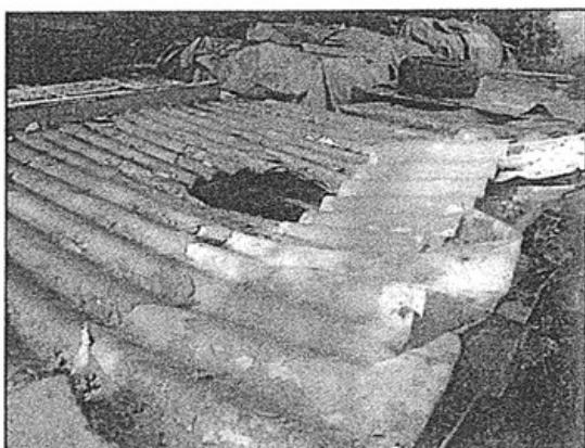
Damaged and holed corrugated sheeting.
