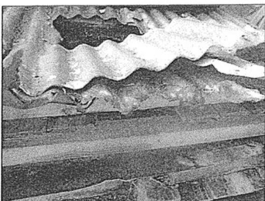
Decayed end of sheeting.
