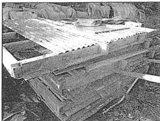
Wall panels stored in bundles.
