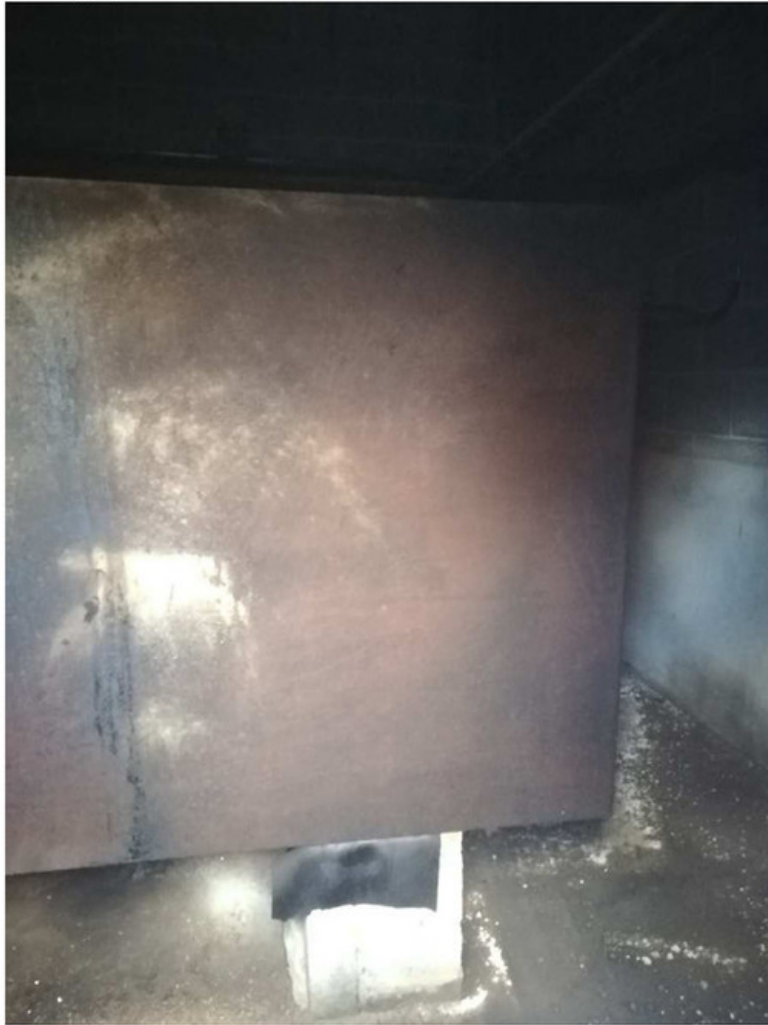
Photograph 3 – OIL STORAGE TANK
