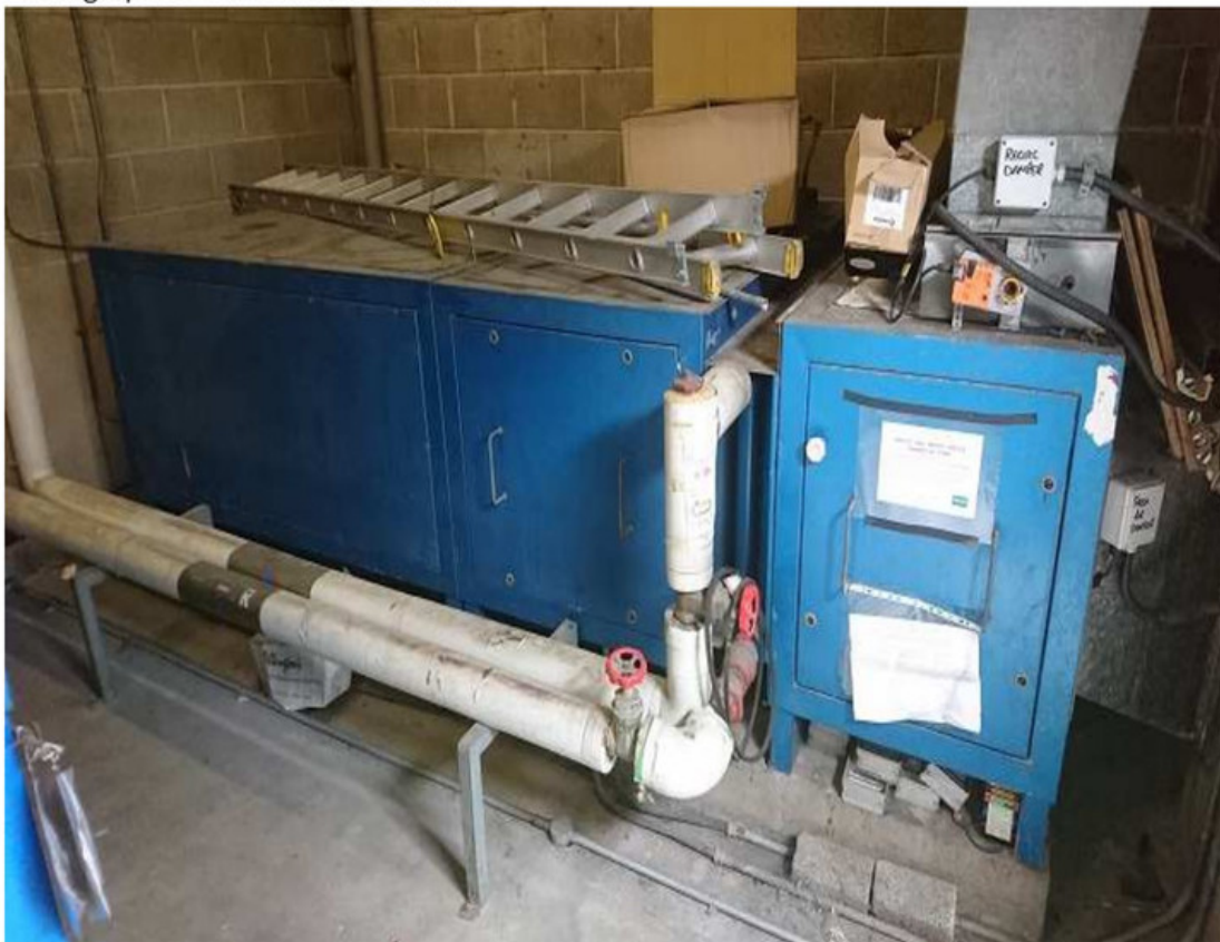
Photograph 6 – AIR HANDING UNIT
