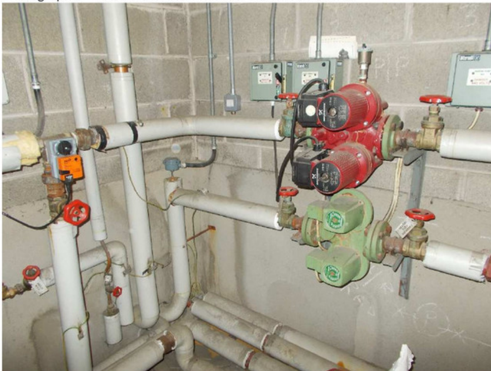
Photograph 8 – RADIATOR AND PRIMARY HEATING PUMPS.
