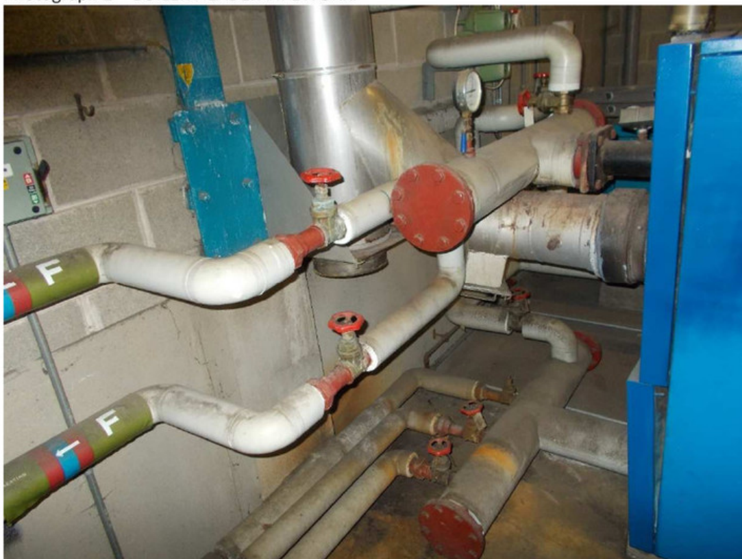
Photograph 2 – BOILER HEADER PIPEWORK.
