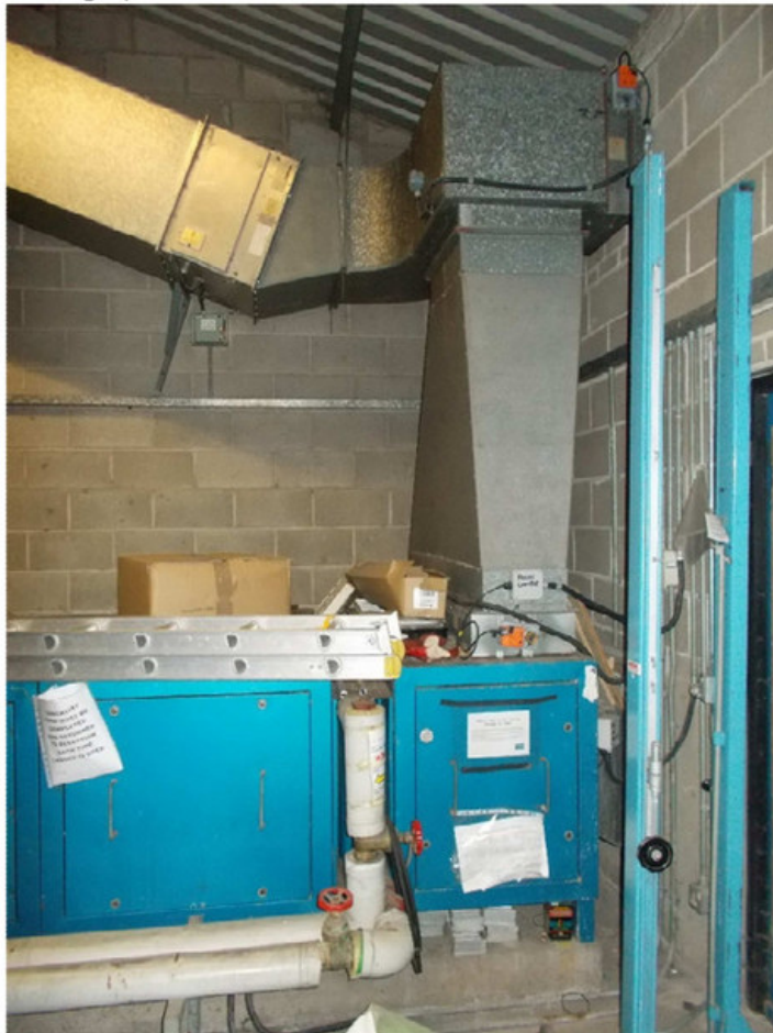
Photograph 7 – RETURN AIR FAN AND MIXING BOX
