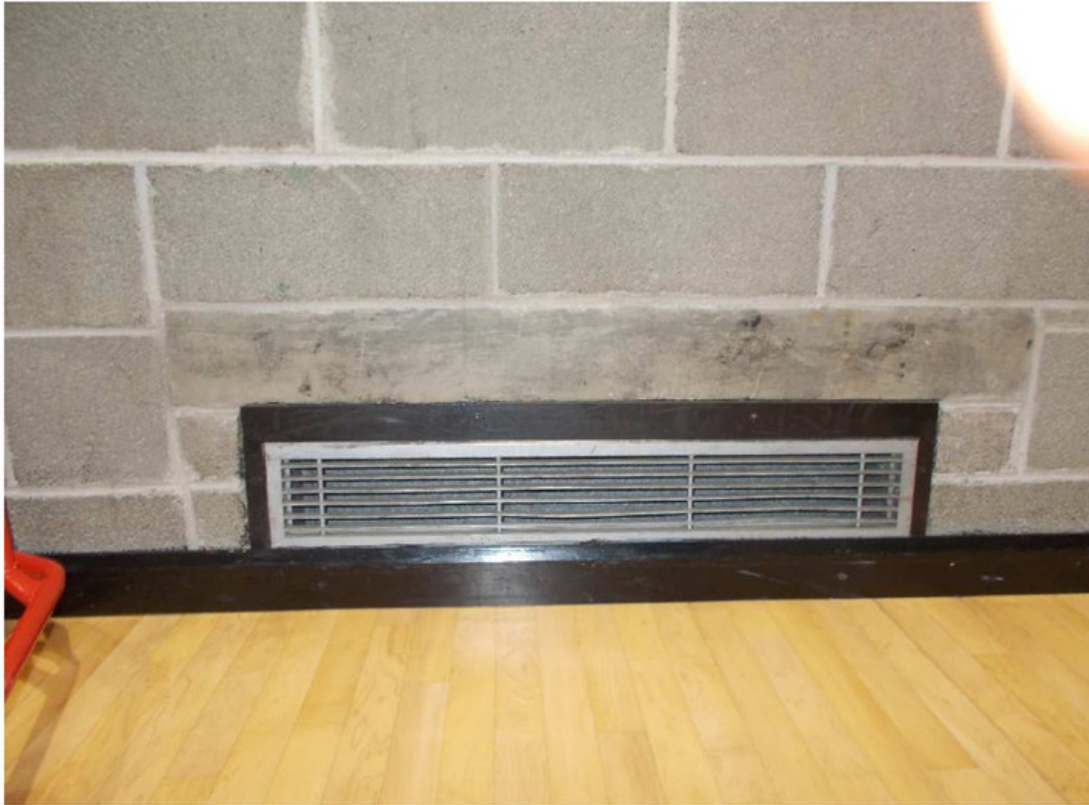
Photograph 5 – LOW LEVEL AIR SUPPLY GRILLE
